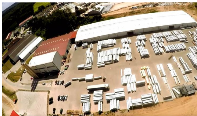
Fig. 1. The view of WITAL plant in Goldap
